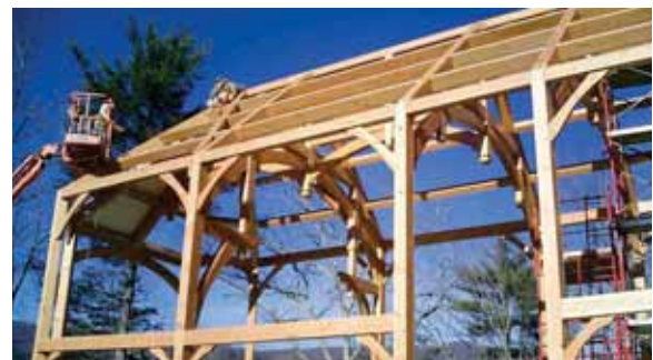
Raising of timberframe
